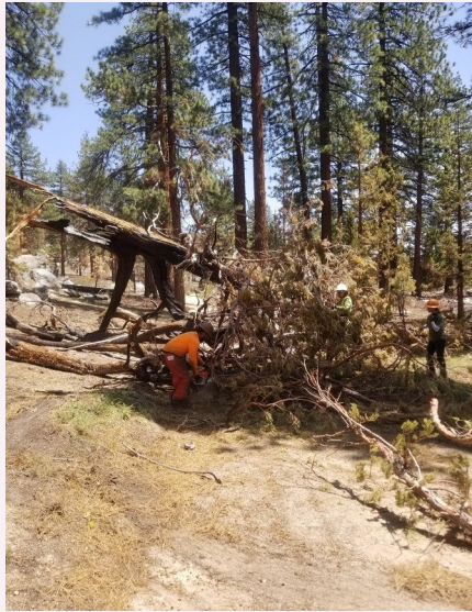
Tree across road being cleared
