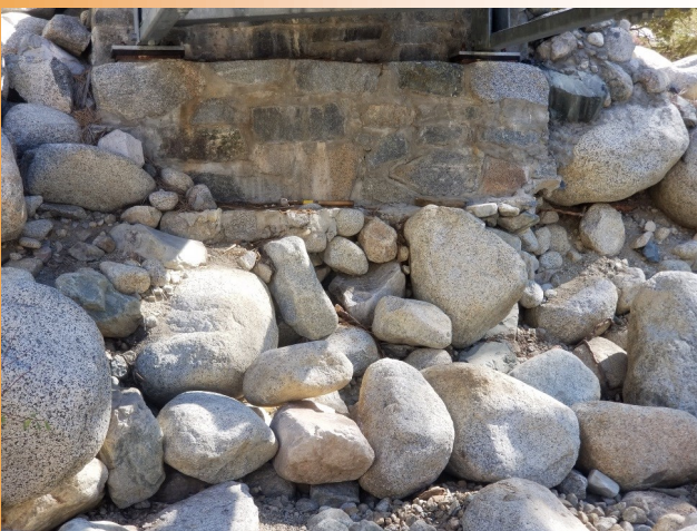
Bridge abutment erosion
