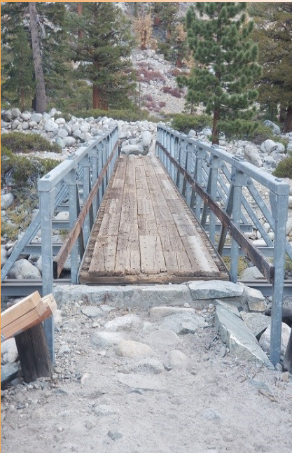
Before bridge repair
