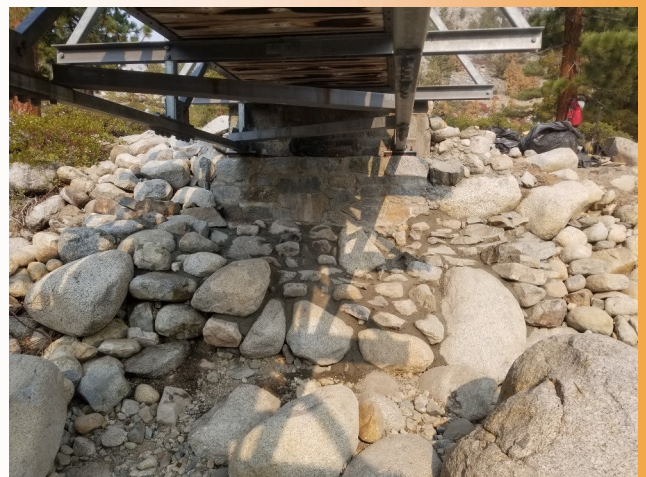
Bridge abutment repaired
